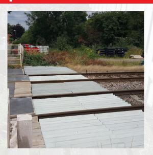
HR Kilns standard and fire retardant Anti Trespass panels are now available for use with most track gauges worldwide. Made from GRP (Glass Reinforced Plastic), our panels have many advantages over other products.
